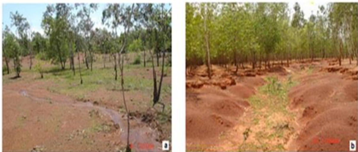
Plate-4:a) A scour networking in afforested gully near Jhargram b) A linear gully drainage at jhargram
